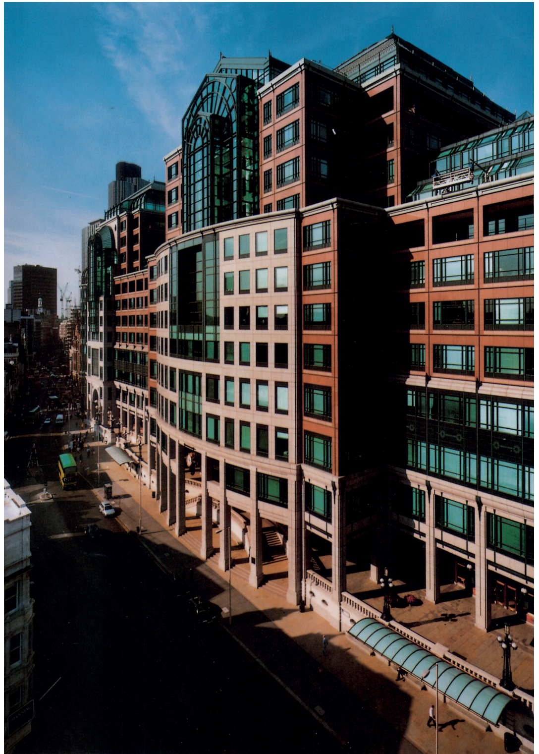
Broadgate's 135 & 155 Bishopsgate blocks are 'PLATTENBAU BEAUX ARTS' - East Germany's answer to Paris. They are built of panels, one storey high and one window wide. Check the black lines. The walls are thin slices of granite glued to a light steel frame. The openings are a big sheet of plate glass decorated by stuck-on 'Chicago' window-bars.
